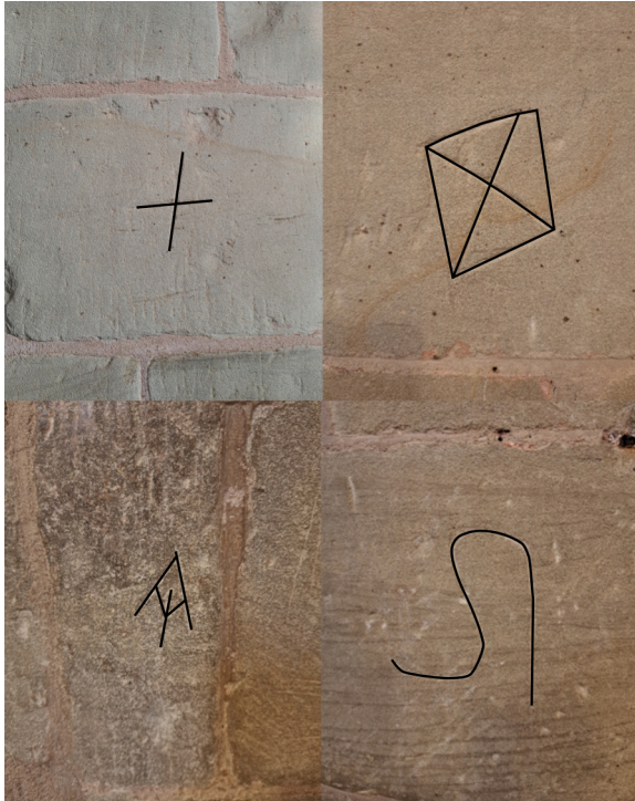
Fig 3: Combined crux quadrata , hourglass, arrow and curvilinear banker marks on the nave piers of Great Malvern Priory (author's photo)
